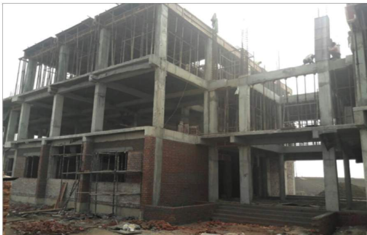
A View of Construction of Building of Central Food Testing Laboratory at Faridabad
