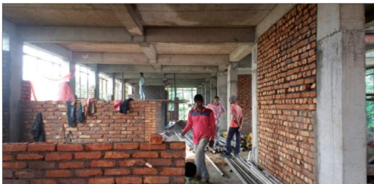
A View of Construction of Building of Regional Food Testing Laboratory at Kolkata
